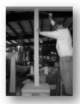
Measure overall opening from floor to beam or soffit (must have structural pressure-treated post or lally column for load-support.
