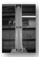
Place the partially assembled (3 panels) column around post and blocking.
