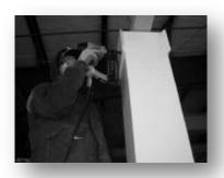
Option 2: Leave 1/4" expansion room above cap, and pin-nail the cap to the column. Be sure pin-nails DO NOT reach the blocking inside!\*
