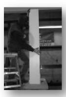
Screw or nail column to blocking ONLY ON THE BOTTOM. Do not attach at center or top (to allow for expansion).
