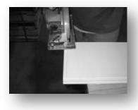
Trim shaft pieces at least 1/4" shorter than opening height (from Step 1). Trim ONLY from the bottom of the shaft – top end is marked.
