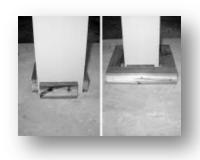
Install blocking around load-bearing post (use pressure-treated lumber). Final width of blocking must be the same width as the inside of the column.
