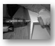
If using screws, assemble three (3) panels together using coarse thread galvanized screws (deck screws).
