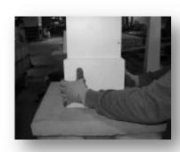
Apply adhesive to mitered ends of base moulding (9-1/4" tall) and assemble around bottom of column shaft.
