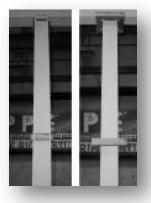
Install blocking around center and top of post to match Step 2. (Center blocking is optional). Blocking may be attached to deck/soffit instead of the post if necessary.
