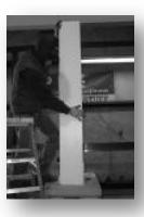
Apply adhesive to final panel and attach to column shaft using the easy interlocking joints.
