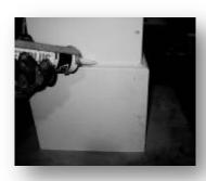
Caulk edges of base, cap, and nail or screw holes.
