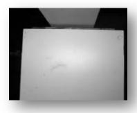
The TOP of the column shaft should NOT be fastened to the blocking, and there should be at least 1/4" gap to allow for expansion (see Step 4).
