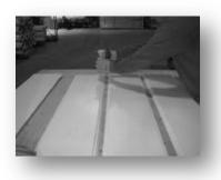
Lay three (3) panels flat and apply adhesive to center joints. (Polyurethane glue is recommended. Follow manufacturer's instructions).
