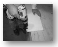
If you are going to use screws, predrill/countersink all panels. See joint diagram on last page to determine which edge to pre-drill.
