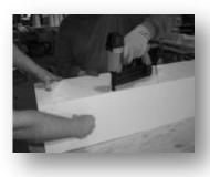
Or if you are not using screws, finish nailing the three (3) panels together.
