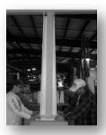
Slide assembled 3-sided column around support (on top of base).
