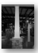
Clean surface of column with cleaner recommended by the paint manufacturer. Paint with two (2) coats of acrylic latex paint.
