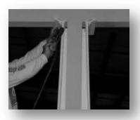
Raise cap to beam/soffit, center, and attach. There should be 1/4" between column and cap platform.
