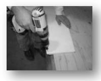
If you are going to use screws, predrill/countersink all panels. See joint diagram on next page to determine which edge to pre-drill.
