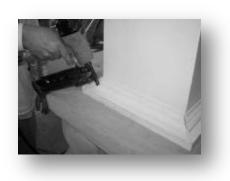
Apply adhesive to moulding and pinnail into place.
