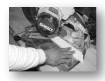
Using miter saw, cut base trim pieces to fit around bottom of column.
