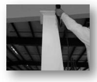
Glue ¼ cap piece and slide into place. Pin nail cap moulding to top of column.\*
