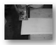
Trim shaft pieces to 2-1/4" shorter than opeing – 2" for cap/base, 1/4" for expansion (1/4" if not using cap & base – each part is 1" thick.)
