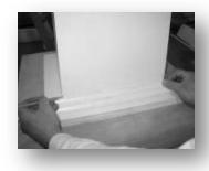
Use column shaft to mark cut lines for miters (cut long and work your way shorter for best results).
