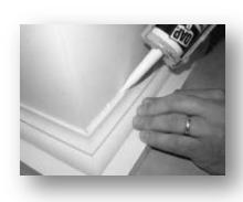
Caulk using latex caulking compound to fill any gaps and nail or screw holes.
