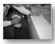
If using screws, assemble three panels together using coarse thread galvanized screws (deck screws).
