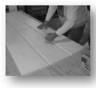
Lay 3 panels flat and apply adhesive to center joints. (Polyurethane glue is recommended. Follow manufacturer's instructions.)
