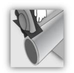
Measure the opening where the column will be installed. When calculating the overall height required, be sure to include the height of the capital. Trim the column shaft from the bottom to fit the height of the opening. (Column may be trimmed with a circular saw that has an abrasive blade.)
