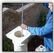
Lower the threaded rod into the column & engage the coupling nut on the bottom.
