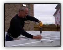
Set the clutch on the drill to insure that the screw head does not dimple the top surface of the purlin.
