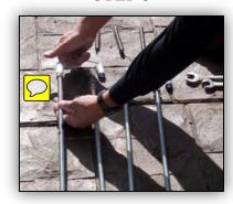
Attach a connector nut to the threaded rods & then attach the short six-inch stainless steel threaded section to the top of the connector nut.
