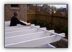
Following the layout pattern on the rafters, begin installing the Purlins across the top of the rafters using the steel deck screws.
