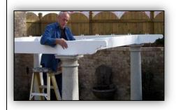
Install the headers with the decorative rafter tails on the opposite side of the aluminum angle using the 2.5" hex head stainless steel self tapping screws. Set the clutch on the drill so the screw is not stripped.
