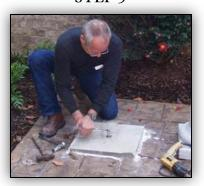
Use the 15/16" socket wrench to tighten the nut on top of the anchor.
