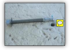
Use the hammer to install the stainless steel anchor in the prepared hole.
