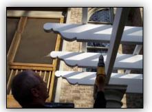
Using a 1/8" drill bit, drill a hole in the bottom near the end of each header, rafter & purlin. This will insure that moisture will vent – should any collect.
