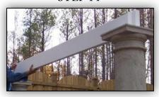
Install headers without decorative rafter tails to outside of the aluminum angles on top of columns using the 2.5" hex head stainless steel screws. Set the clutch on drill so the screw is not stripped.
