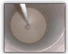
Screw the threaded rod snugly into the coupling nut at the bottom of the column & tighten with pliers.
