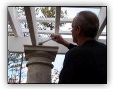
Using a 15/16" deep well ratchet or opened end wrench, tighten the nut on top of each column until very tight.
