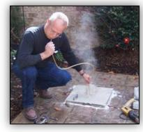
Remove the dust from the hole to insure a clean insertion of the stainless steel anchor.
