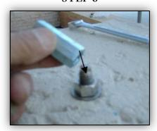
Install the connector nut on top of the stainless steel anchor and tighten.
