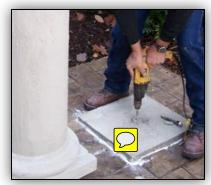
Use the hammer drill and 5/8" concrete bit to drill a five (5) inch deep hole.
