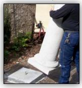
Position the column so that it is centered over the connector nut. If the column base is not installed, slide it over the top of the columns & down the column to the bottom.
