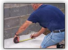
Locate the center points of the Columns. Make sure the layout is Squared. Also make sure the slab is level.
