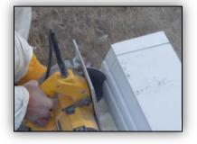
Measure distance between the newel posts and adjust the length of the bottom rail. Use a masonry blade to cut off excess length allowing a 1/8" gap at each end.
