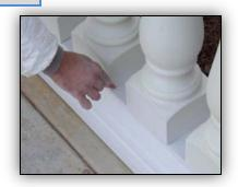
Mark the position of the balusters on the bottom rail with a pencil creating a reference point.
