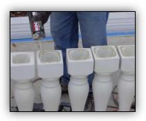
Put adhesive on the bottom edge of the balusters.
