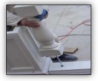
Place balusters over threaded rods and in the position you marked with pencil, previously. Position remaining balusters as marked.
