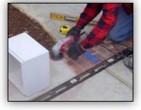
The base must be level. Therefore, it may be necessary to level the surface upon which the system will be installed by grinding (if possible). You may need to cut off some of the bases well to insure that it is level.
