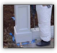
Be sure rods are securely placed in the anchors.
