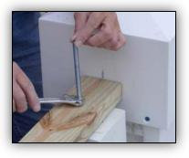
Position the "2 x 4" over the threaded rods and use a washer and hex nut to snug the "2 x 4" into place. DO NOT over-tighten. Cut off any excess rod length.
