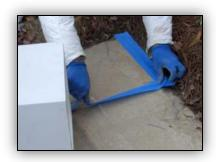
Place tape around the edge of the pencil marks to protect the surrounding surface from excess glue.
