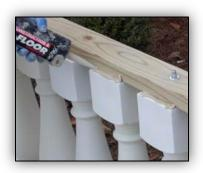
Put adhesive on top edges of baluster not covered by the "2 x 4".
