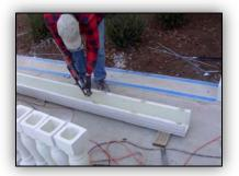
Drill holes through the bottom rail as marked. Spot glue every 18" on the bottom rail.
