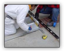
Once the base is level and in position, mark the placement by penciling around the outside edge.
