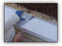
Find the center of 4 equally spaced balusters per each 10' section for placement of threaded rods. (Refer to installation instructions.)
