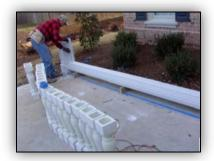
Tap concrete to mark corresponding placement of the anchors and rods. Move rail and install anchors and rods.
