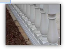
Line up all balusters with the bottom rail with the seams all facing in the same direction. You may need to adjust the number of balusters to meet the 4" code requirement; or, to insure equal spacing if not.
