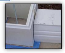
Temporarily place bottom rail in position, using shims to steady.
