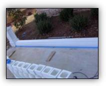
Mark placement of bottom rail with pencil and tape to prevent excess glue runoff.
