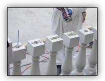
Spot glue top of balusters on which the  $^{\circ}2 \times 4^{\circ}$  will be placed.
