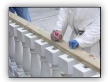
Place the treated "2 x 4" on top of the balusters marking the center position of the rods. Drill a ½" hole for the rods to come through.
