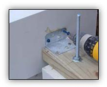
Center the "L" bracket on the "2 x 4" and screw into place.
