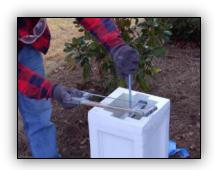
Cut off the excess length of the threaded rod.
