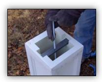
Install the channel iron and secure with the hex nut.
