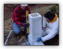
The center section of the columns must be level; if it is not, refer to the installation instructions for leveling of the newel post.
