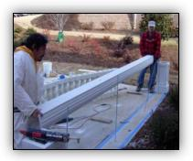
Lift bottom rail and place it into position over the rods.
