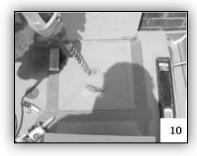
As decking is not solid enough to provide adequate support, it is necessary to reinforce the rod.
