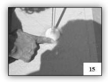
Holding rod upright, tighten the nut. Be careful not over-tighten the nut.
