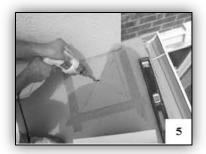
Drill a ½" or 5/8" hole for the placement of the wood insert. The hole size depends upon the size of the wood insert & rod sent with your hardware.
