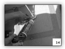
Place a generous amount of silicone between the gasket material and the bottom of the fender washer.
