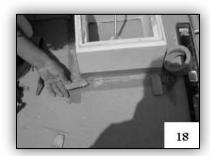
Use wooden shims if necessary to level the base.
