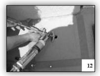
Place a 3/8" hex head nut on the rod, a 2" fender washer, the gasket material and then a 3/8" butterfly nut.
