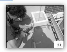
Flush cut the shims to edge of base and apply silicone to fill in the gaps and secure the base. Leave some room for the painter to apply caulk.
