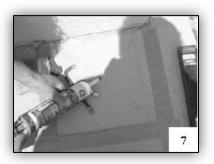
Fill hole with best quality silicone before positioning the insert.
