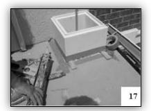
Apply adhesive to bottom of base and position within taped area.
