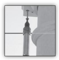
Apply construction adhesive to top of capital, press against structure, and screw or nail into place. Use a nonacetone based exterior grade construction adhesive. **STEP 8**
