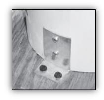
Mark and drill holes in floor and column shaft for corner/angle brackets (not included).
