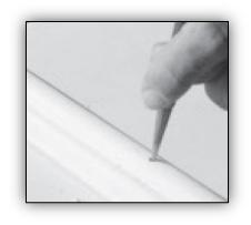
Set screws or nails and use caulk to cover the holes.
