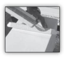
Pre-drill holes through neck mold into column. Screw neck mold in place or pre-drill and use finish nails.
