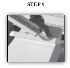
Mark location for supplied neck molding to a 45° angle. Apply construction adhesive and put neck mold in place. Use a non-acetone based exterior grade construction adhesive.
