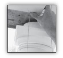
Put assembly in place and plumb. Make sure load is centered over the column shaft and evenly distributed around the bearing surface.
