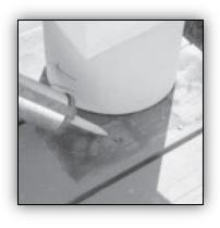
Apply construction adhesive to top and bottom surfaces of column. Use a non-acetone based exterior grade construction adhesive.
